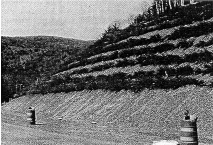
Figure 4. Brushlayer buttress fill immediately after construction. Winter 1990. Greenfield Rd., nr. Route 112, Colrain, Mass.
