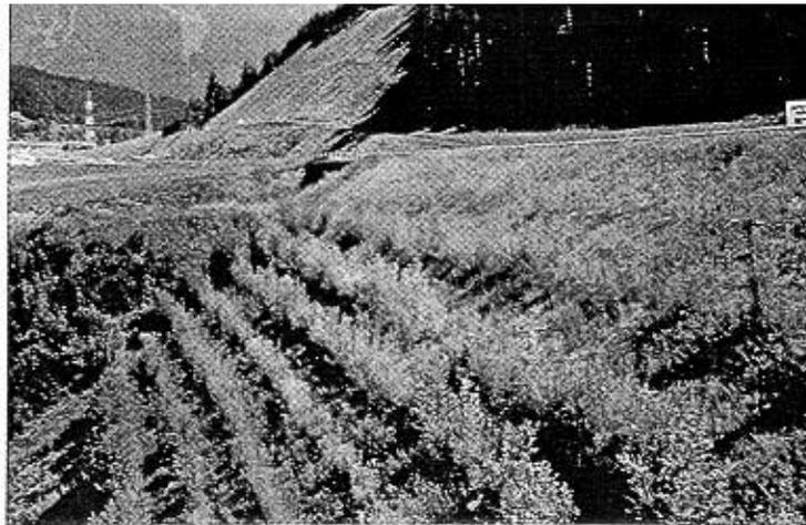
Figure 7. Brushlayer embankment fill stabilization after two years showing both grass and brush establishment. Brenner Pass highway, Austria.
