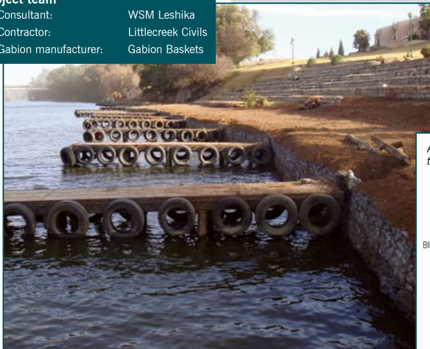
Construction of the Riviera Villas gabion riverbank stabilisation structure.
