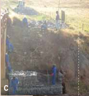
A-F: Construction sequences showing gabion wall and mattress construction in progress on a river diversion and bridge abutment protection project in Kestell in the Eastern Free State.
